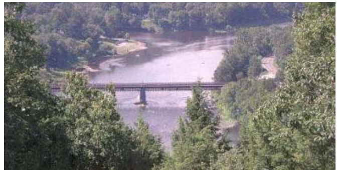
View of the Roebing Bridge at the confluence of the Delaware and Lackawaxen Rivers.
