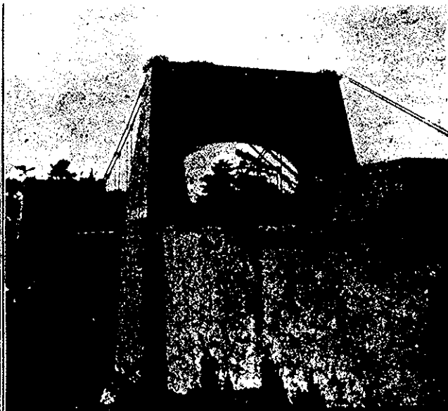
FIGURES 53.—Essex-Merrimack Bridge near Newburyport, Massachusetts, before and after. In the 1909 "rebuilding" of the 1810 structure, the entire superstructure was replaced with a loose replica, leaving of the original fabric only the pier masonry below deck level. (From Engineering News (25 September 1913), volume 70, page 585.)
