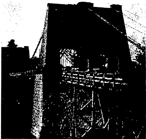
FIGURES 53.—Essex-Merrimack Bridge near Newburyport, Massachusetts, before and after. In the 1909 "rebuilding" of the 1810 structure, the entire superstructure was replaced with a loose replica, leaving of the original fabric only the pier masonry below deck level. (From Engineering News (25 September 1913), volume 70, page 585.)
